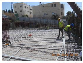
Post tension slab works in Basement -1 Block 1, May 2019
